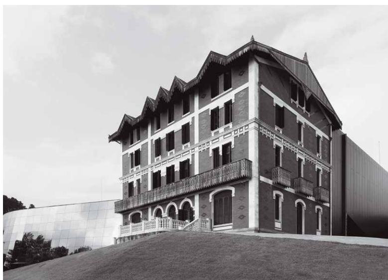
Exterior view of the Cristóbal Balenciaga Museum in Getaria © Cristóbal Balenciaga Foundation / Idoia Unzurrunzaga
